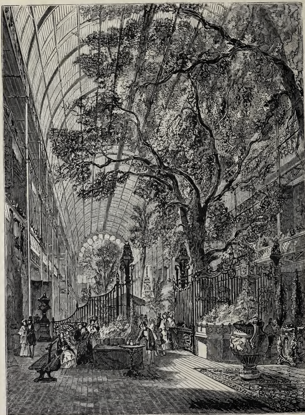
The Transept of the Exhibition of 1851, from the North Side.
